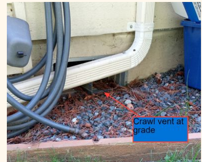
Crawl vent at grade.
