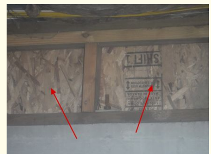
Uninsulated wall framing.
