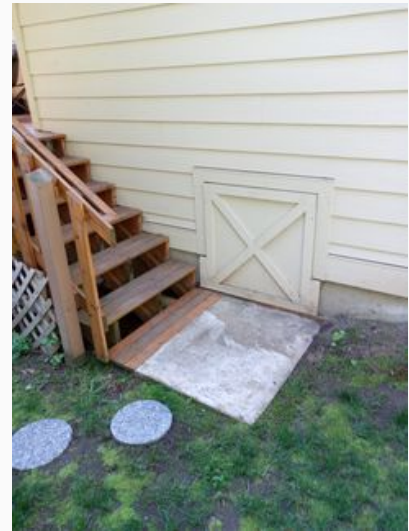
Crawl space access at back of house.
