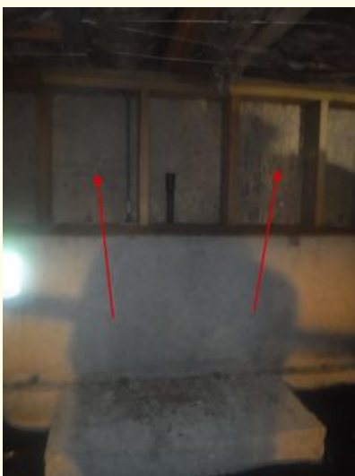
Uninsulated wall framing.
