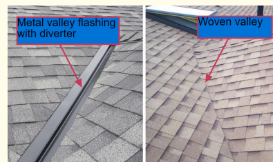
Examples of metal valley flashing and woven valley.
