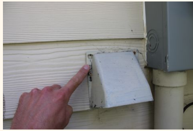
Cracked dryer vent termination with no mounting block.
