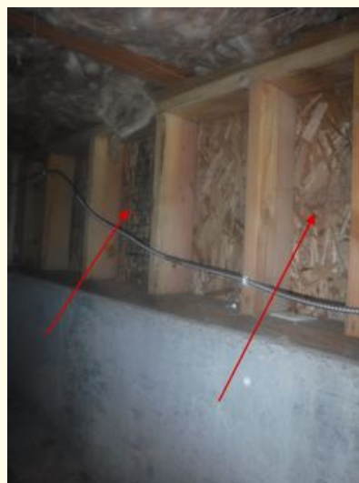
Uninsulated wall framing.
