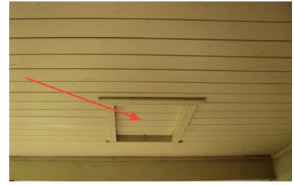
Attic access hatch above back deck.
