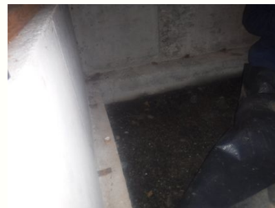
Gravel installed under vapor barrier.
