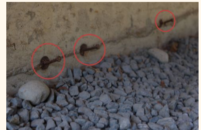
Metal form ties.
