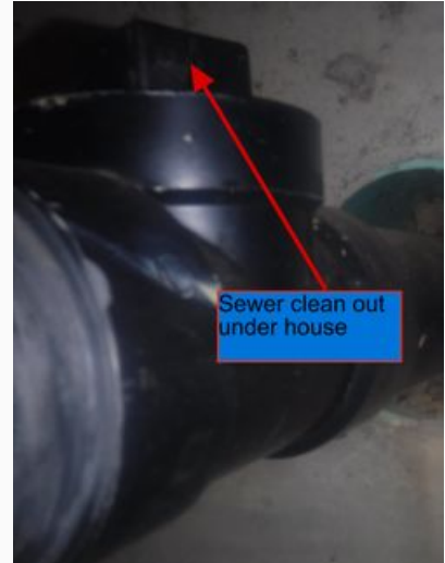
Sewer clean out under house.
