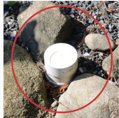
Clean out in side yard.
